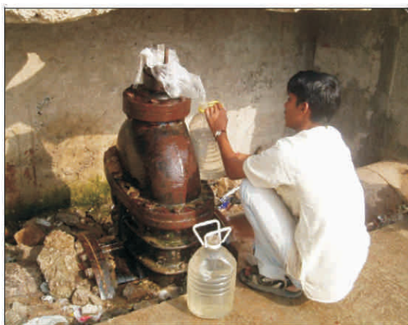
Fig. 8: Leakage of water due to the gland packing
