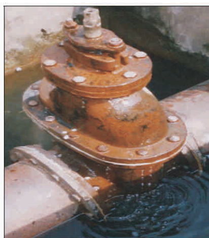
Fig. 8: Leakage of water due to the gland packing
